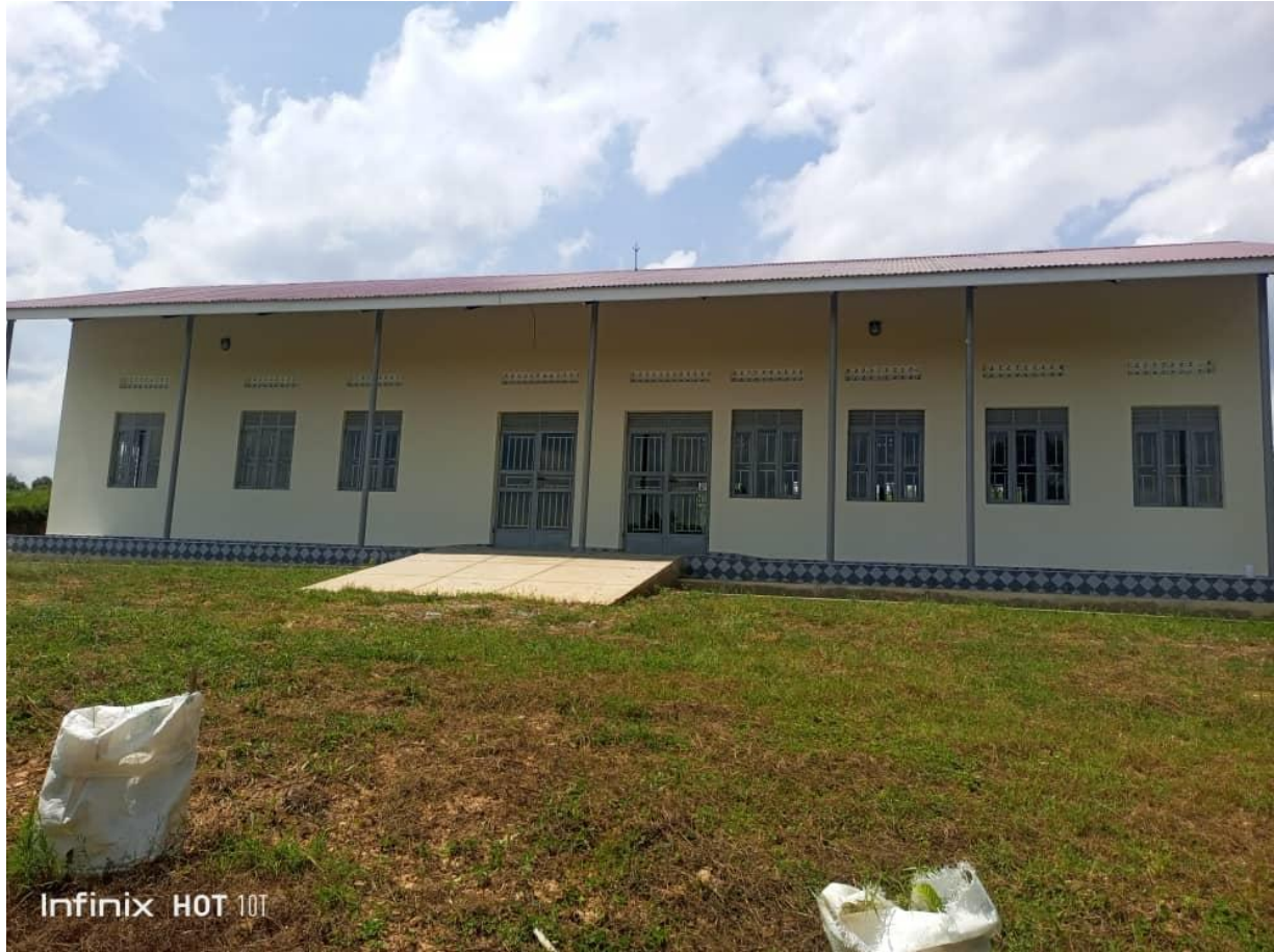
A newly constructed maternity ward at Nyamiko HCIII- Bushenyi ishaka MC
