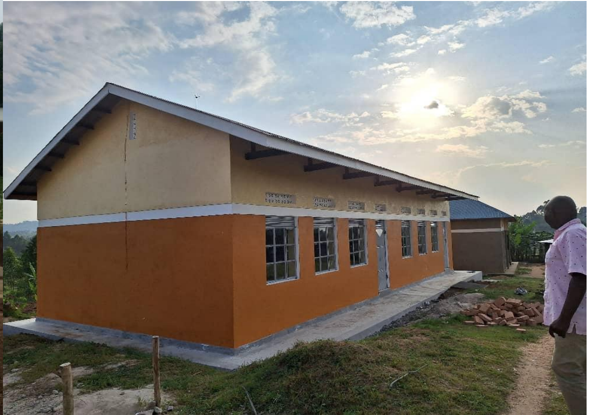
A newly constructed classroom block at Nyakabirizi ps- Sheema District
