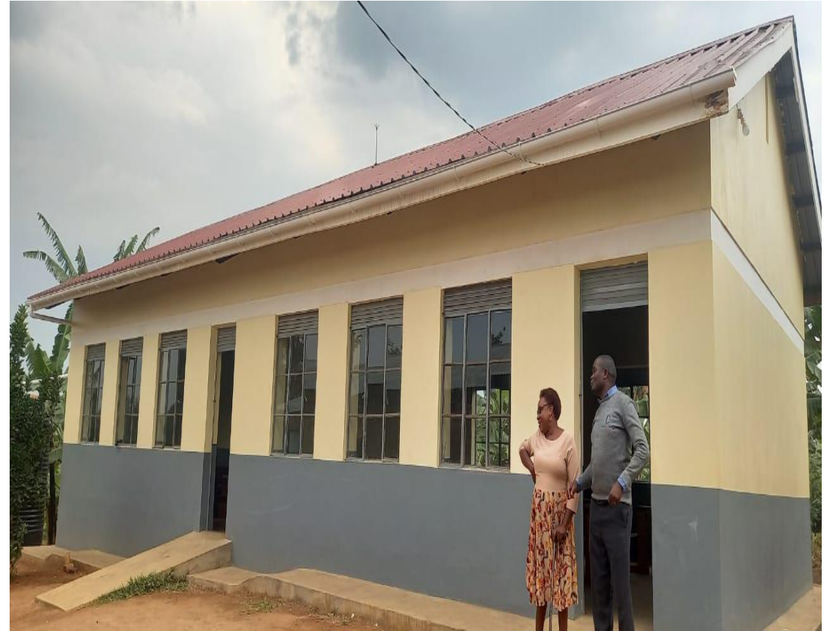
A newly constructed Classroom Block At Kihunda P/S – Sheema MC
