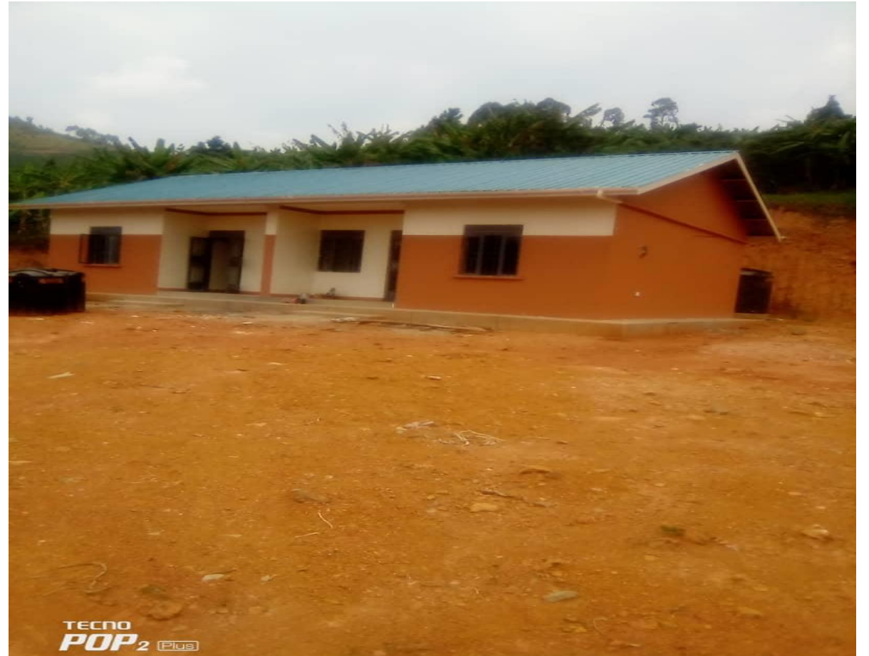
A Newly Constructed staff house at Iyanja HC III in kyahenda subcounty- Buhweju District
