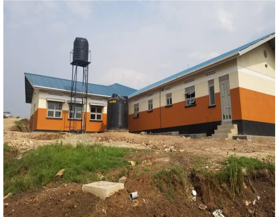
A newly constructed Mwongyera HC III Katerera SC- Rubirizi DLG
