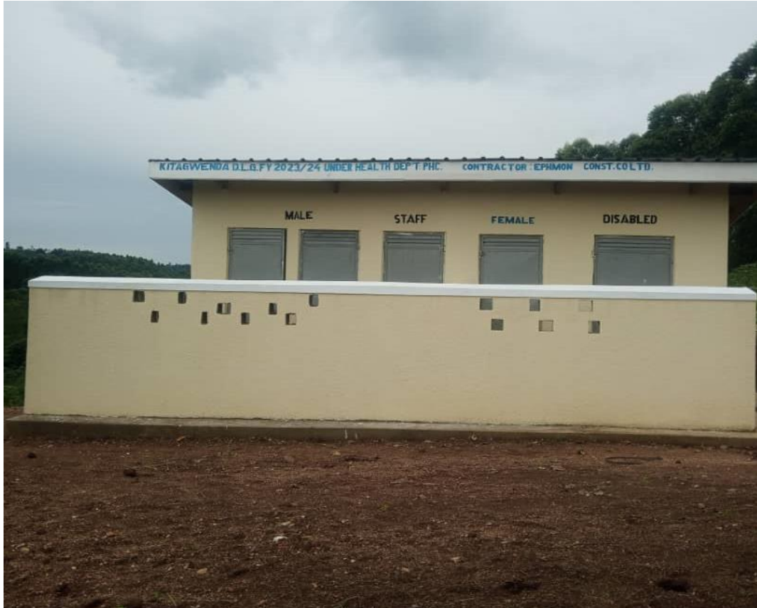
Construction of pit latrine at Kakasi H/Cii, Kitagwenda DLG
