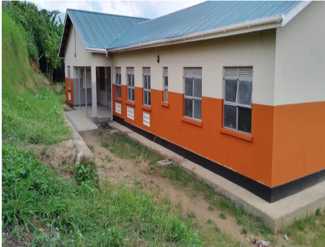
Newly Constructed Mirambi HCIII- Bundibugyo DLG
