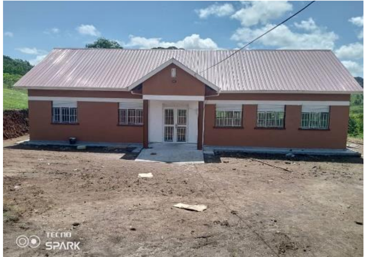
A newly Constructed maternity ward including electrical installation at Migongwe HC II in Kyegegwa District
