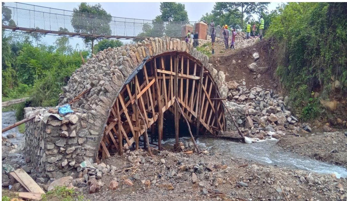
Ntahya Bridge on Bundimwendi- Hakitara road under Construction. The bridge was just during this rainy season. A new arch bridge is under construction.
