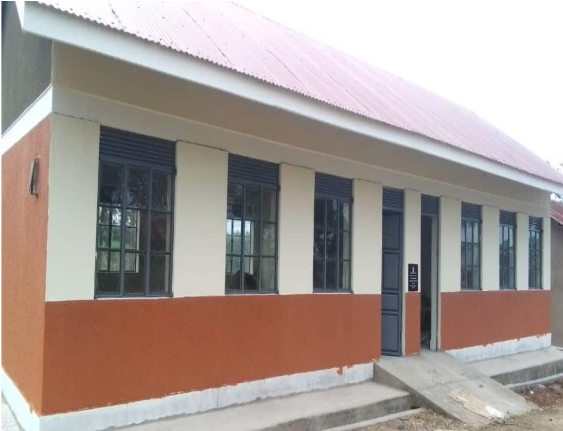
Two Newly Constructed classroom block at Kashaka P.S- Mbararr District
