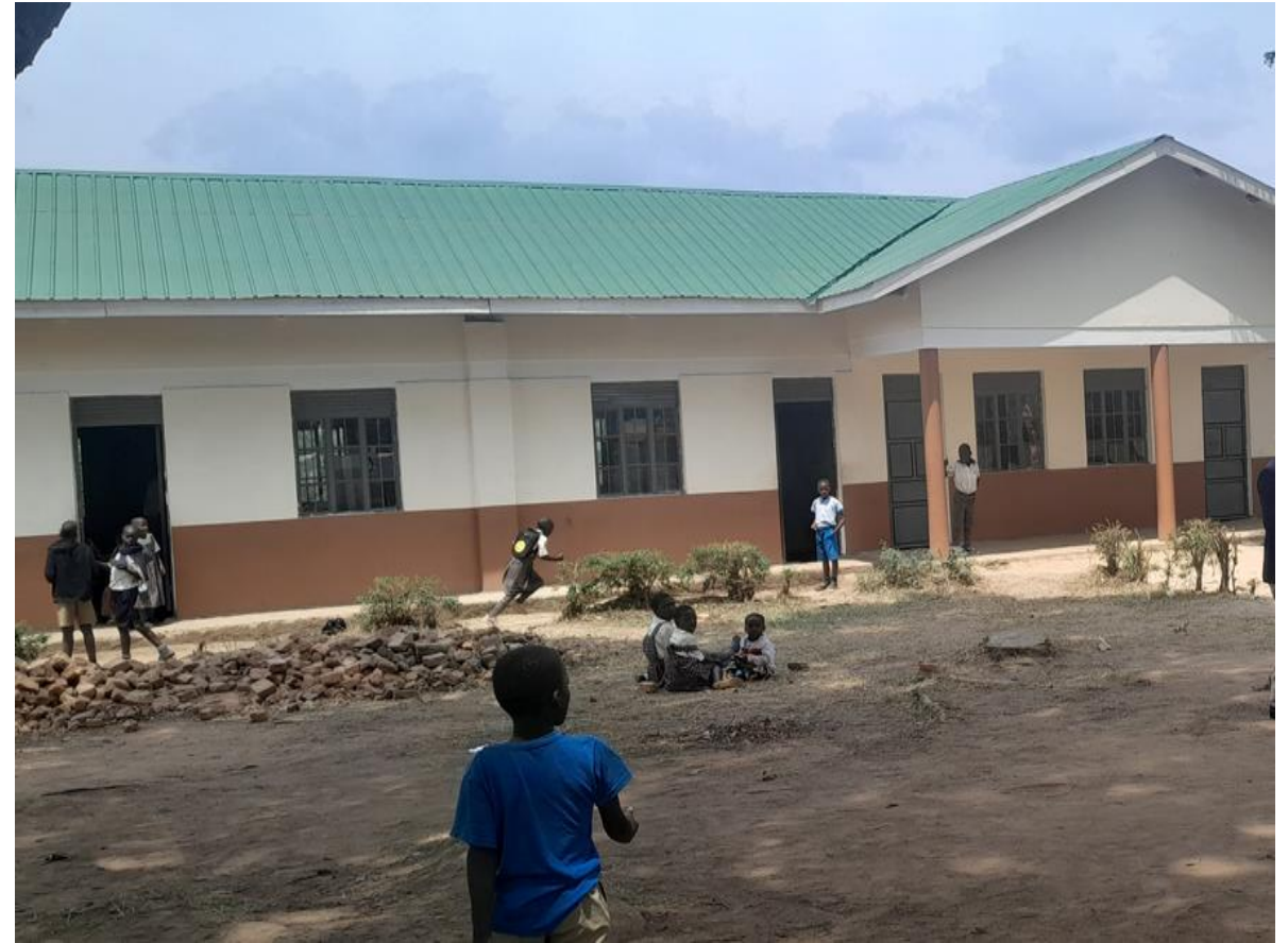
A newly Constructed classroom block at Katukuru PS-Mbarara City
