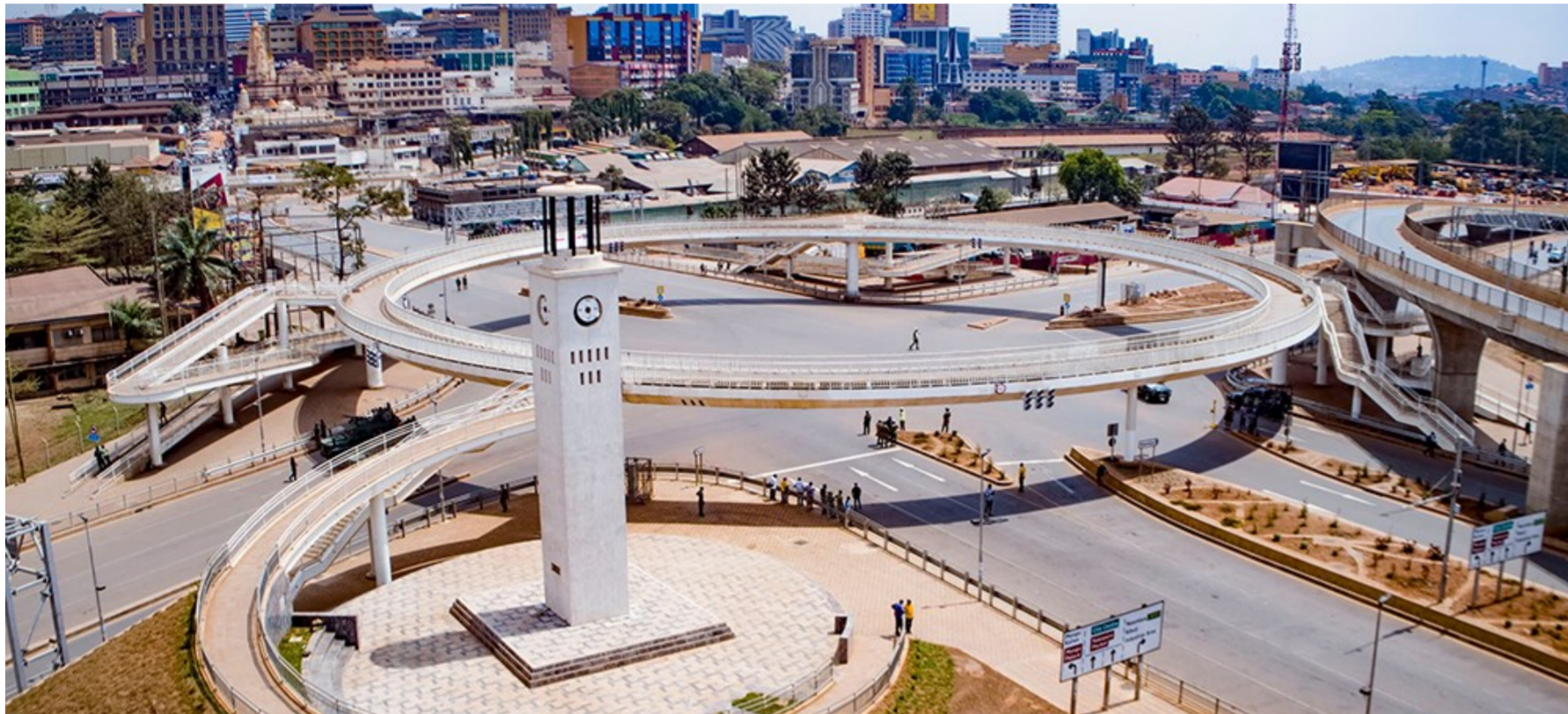
Kampala Flyover Project. Photo: PPU
